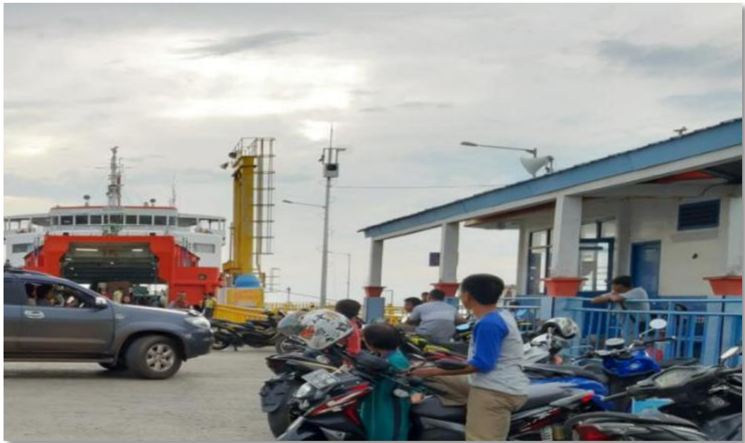
Figure 1. The existing condition of the gangway (Gangway is not connected to sideramp).
