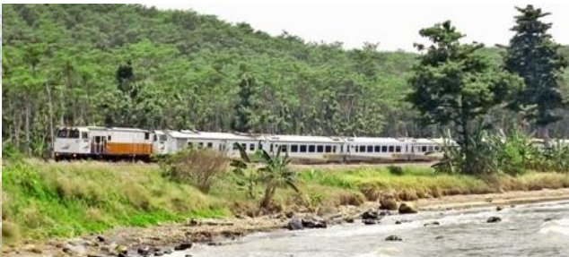
Soil Reinforcement for Railway Structure at Beach - BTIPDP -
